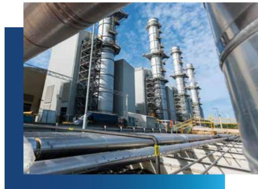
Pembroke natural-gas-fired power station is a gas-and-steam combination power station. A gas turbine serves as a heat source for a downstream waste-heat boiler, which in turn acts as a steam generator for the steam turbine.
